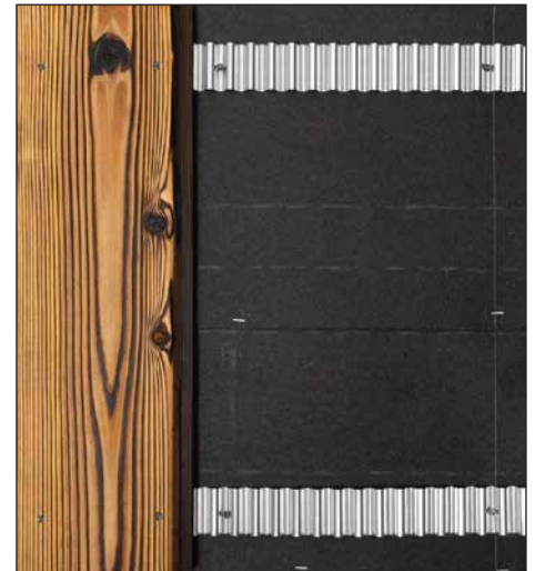
Vertical siding rainscreen installation example
