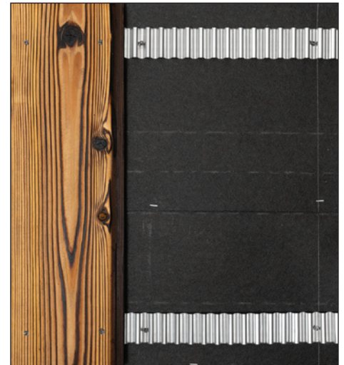
Vertical siding rainscreen installation example
