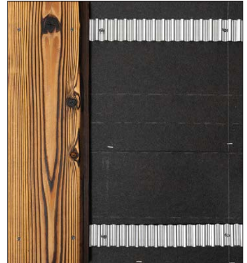
Vertical siding rainscreen installation example
