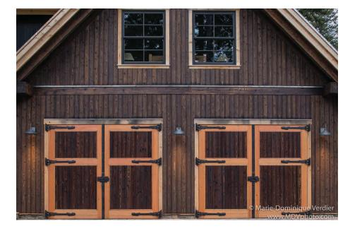
Yakisugi "shou sugi ban" siding and paneling. Wire-brushed, textured surface, with all loose soot removed revealing a striped pattern. Suitable for exterior and interior applications. Available with factory oil prefinish only. Delivered ready to install.
