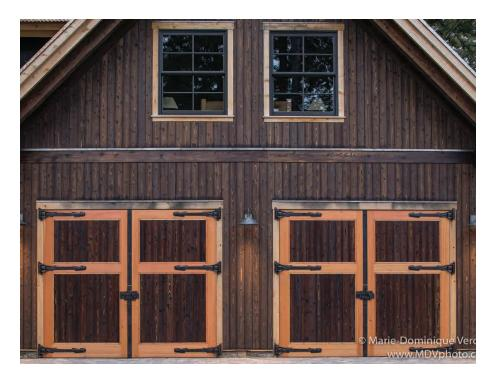
Yakisugi "shou sugi ban" siding and paneling. Wire-brushed, textured surface, with all loose soot removed revealing a striped pattern. Suitable for exterior and interior applications. Available with factory oil prefinish. Delivered ready to install.
